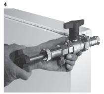
Introduce the stem of the "Demo-Bloc" until it clicks into position. Unscrew the valve insert and pull back the stem slowly until stop.
