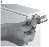
Where space is limited or where radiators are inside a casing, screw the attachment of the "Demo-Bloc" onto the valve first.
