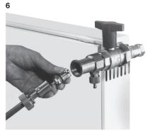
Loosen the inner cap of the "Demo-Bloc" and remove the valve insert for replacement or cleaning.
